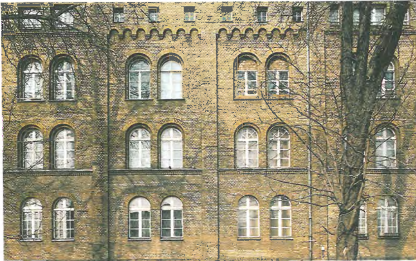
10.1 1860–62 Spandau Grunewaldstraße 8 Garderegiment-Kaserne Fleischinger
